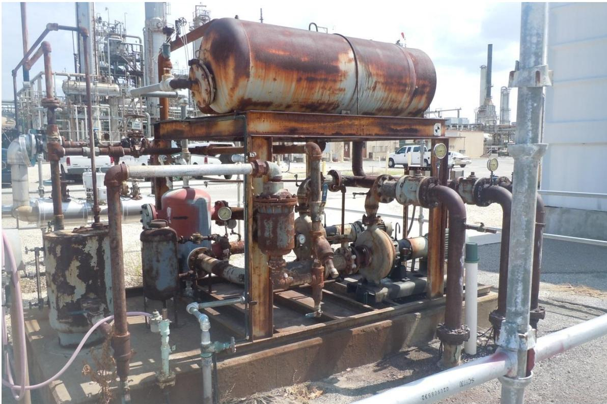
Figure 1: Site photograph of existing hot water skid to be replaced
